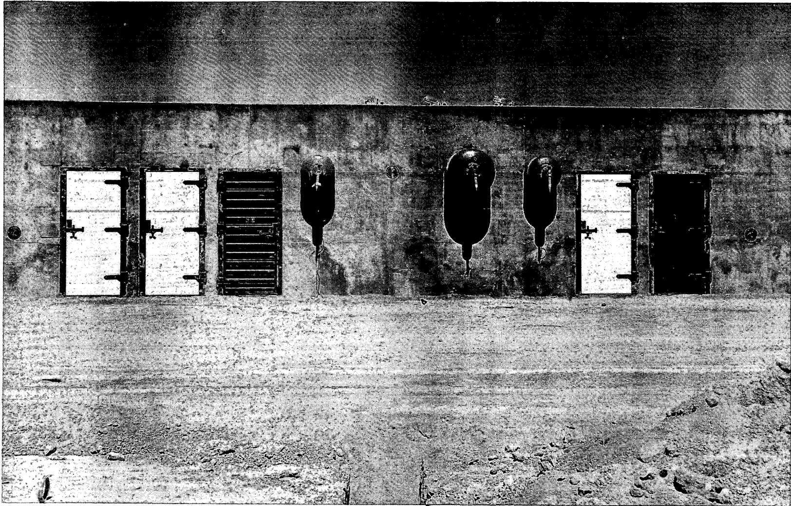
Fig. 8—Typical cell closures. Doors, from left: solid plywood, wood plank, cellular steel, hollow plywood, and steel plate.
